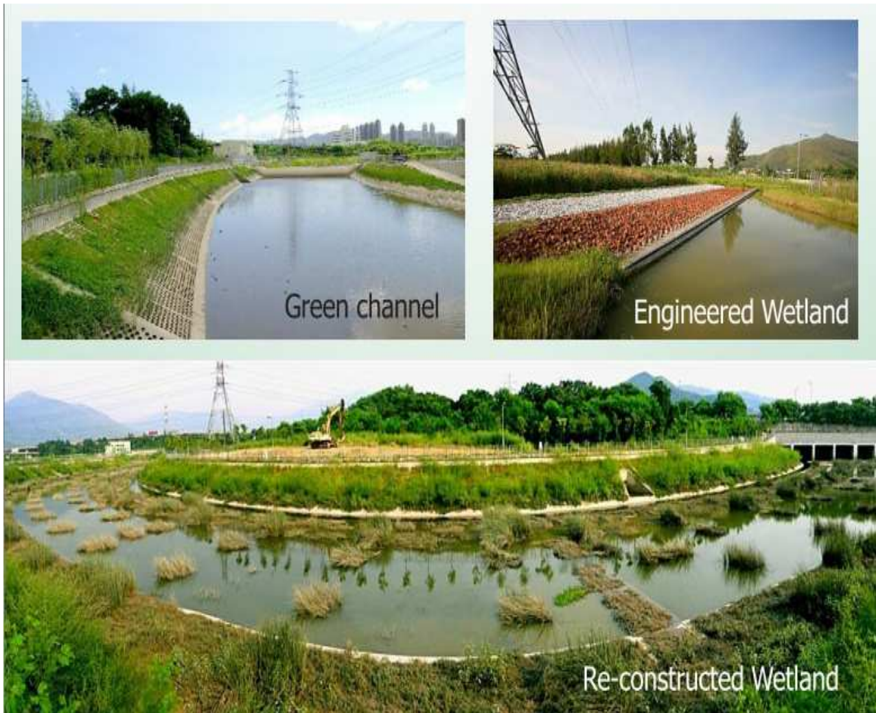
Fig.4 Green Flood Prevention System in Hong Kong
