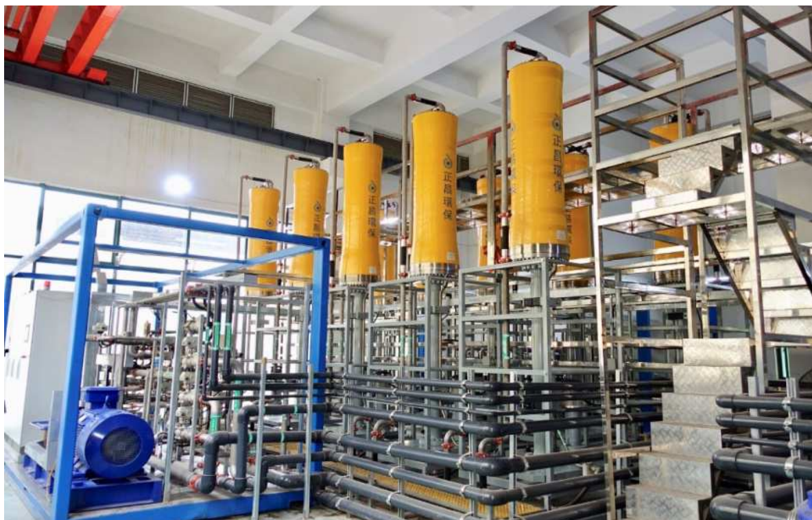
Fig.8 ZLD Pilot Plant for Coal Gasification in China
